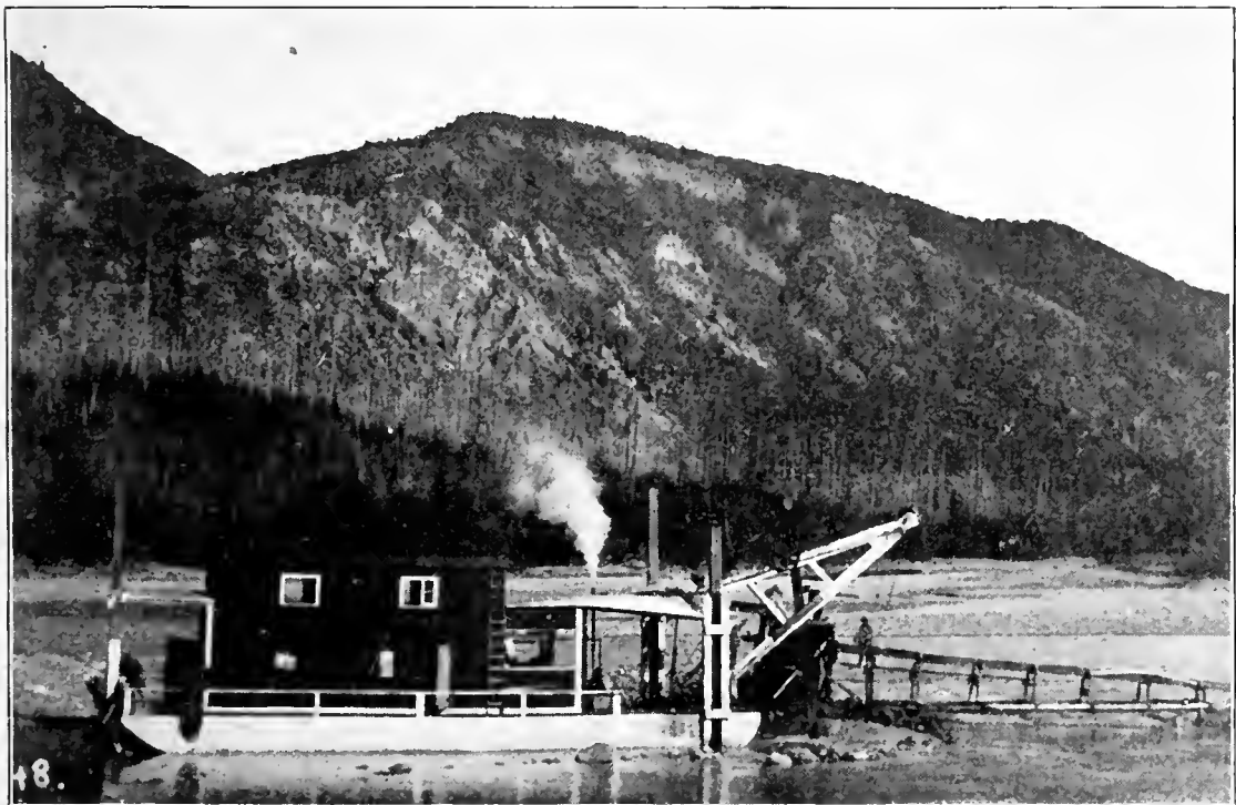
NEWALL DREDGE—IN OPEN WATER.
